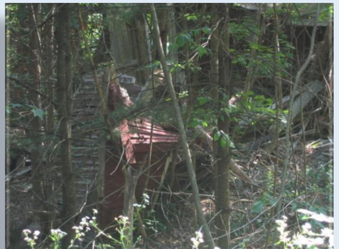
Remaining ruins of Old Man Brown's former home.
