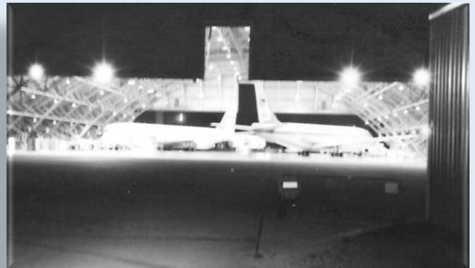
The hangar at night with doors opened on both ends, #26000 and one of the other three parked inside
